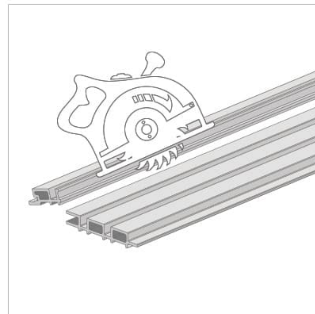
04. Cut the wall panels to fit the remaining length.
